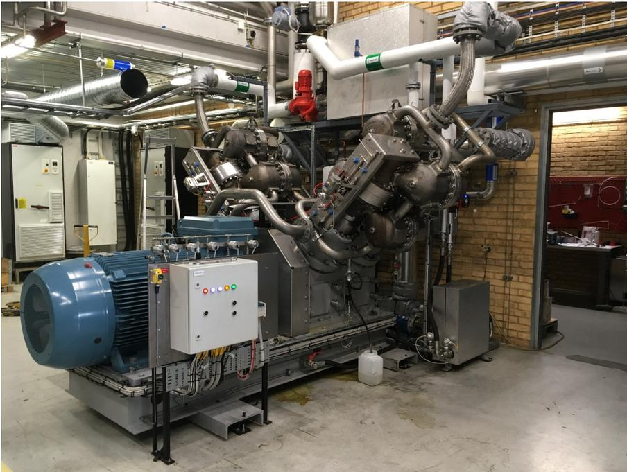
Figure 7. The HighLift HTHP from Olvondo Technology installed in the heat pump room at AstraZeneca, Gothenburg, Sweden. The nominal heat output from the heat pump is between 450 and 500 kW.
