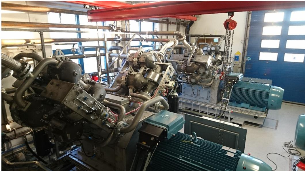
Figure 3. Two of three Highlift HTHP heat pumps from Olvondo Technology installed at the dairy plant used in this example. The heat pumps are replacing steam generation by natural gas fired boilers.
